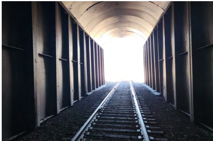
Segment 6 overall view upstation
