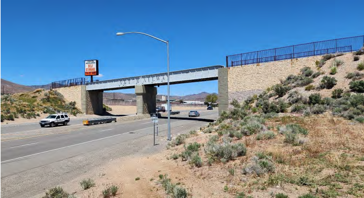
VTRW Bridge Facing East along Eastbound Highway 50
