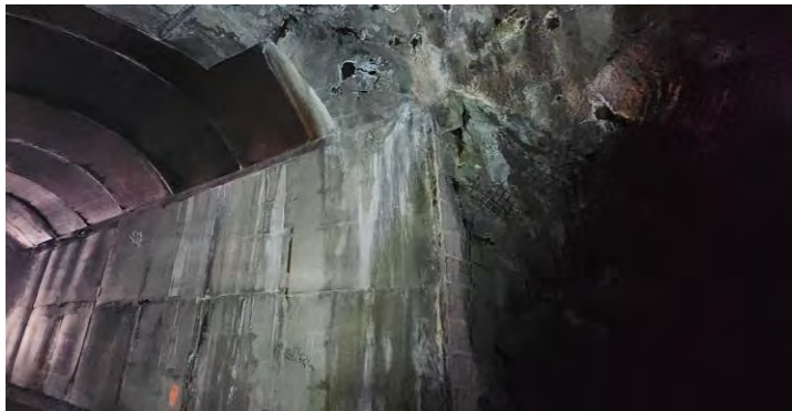
Transition from Segment 3 to 4
