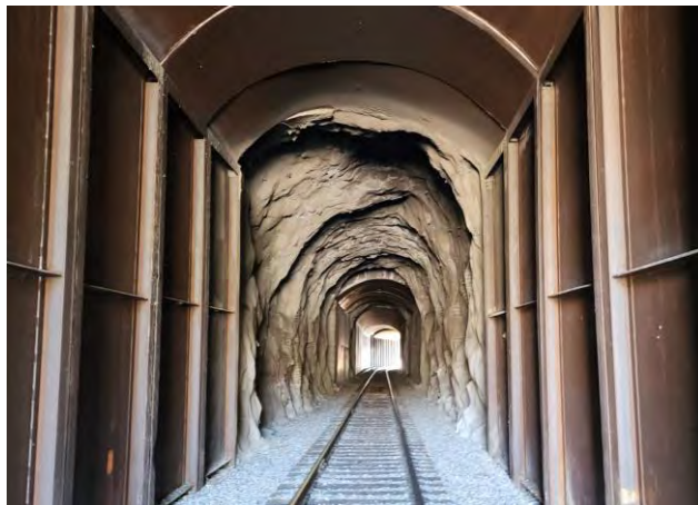
Transition from segment 6 back to 5 (downstation)
