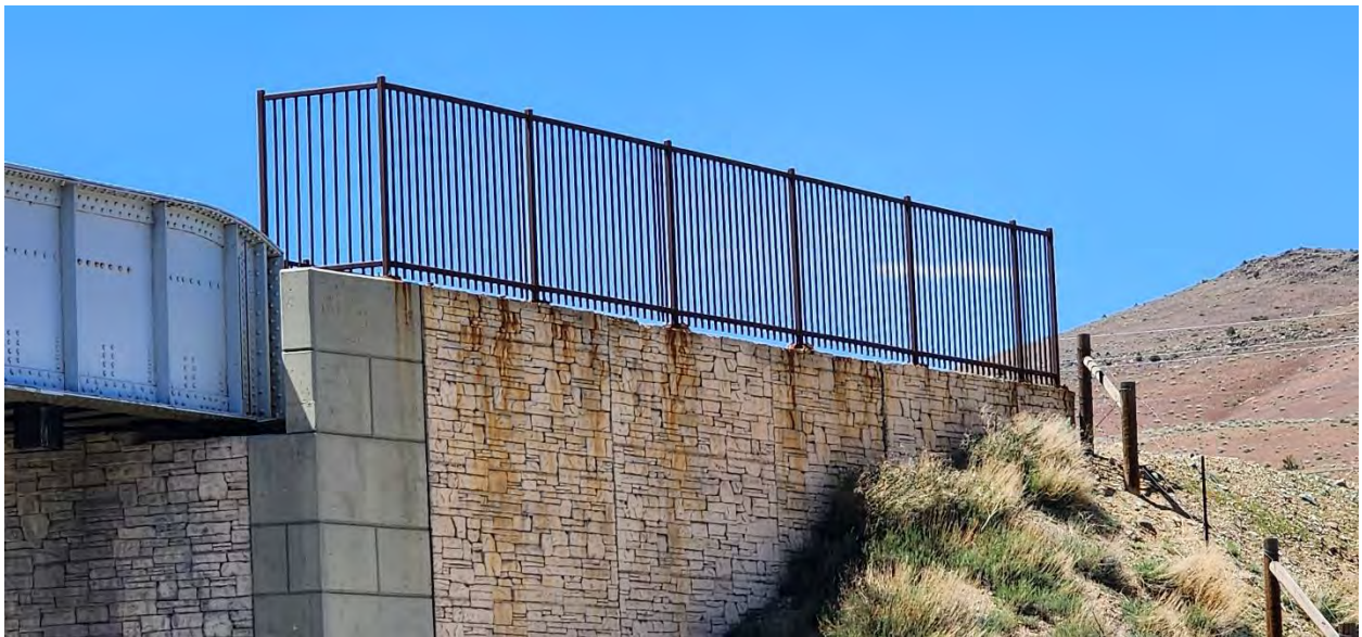
North Abutment East Wingwall Facing Northwest
